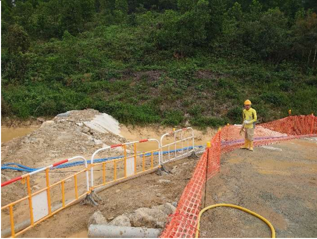
Sedimentation basin at Portion E4
