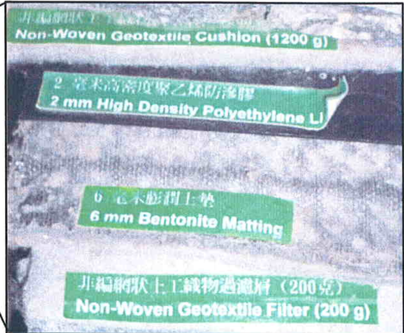
Cross-section of lining and leachate collection system
